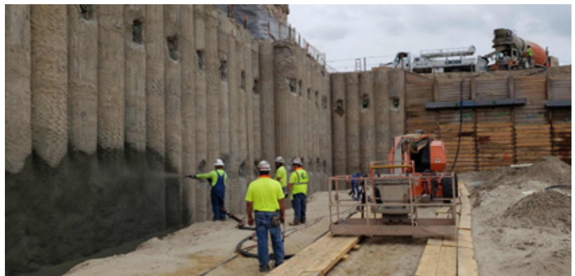
Applying Shotcrete to the Secant Wall
