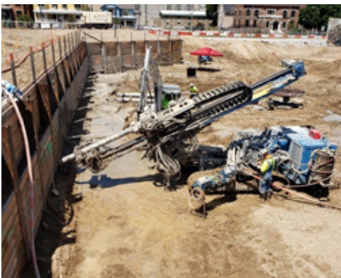
Tieback Installation
