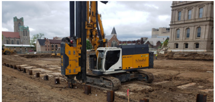
Installing the Secant Wall Several Feet from the Capitol Building
