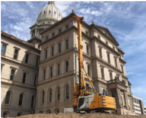
Bauer BG-26 Drill Rig
